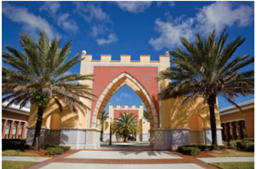
Community Building Entrance
