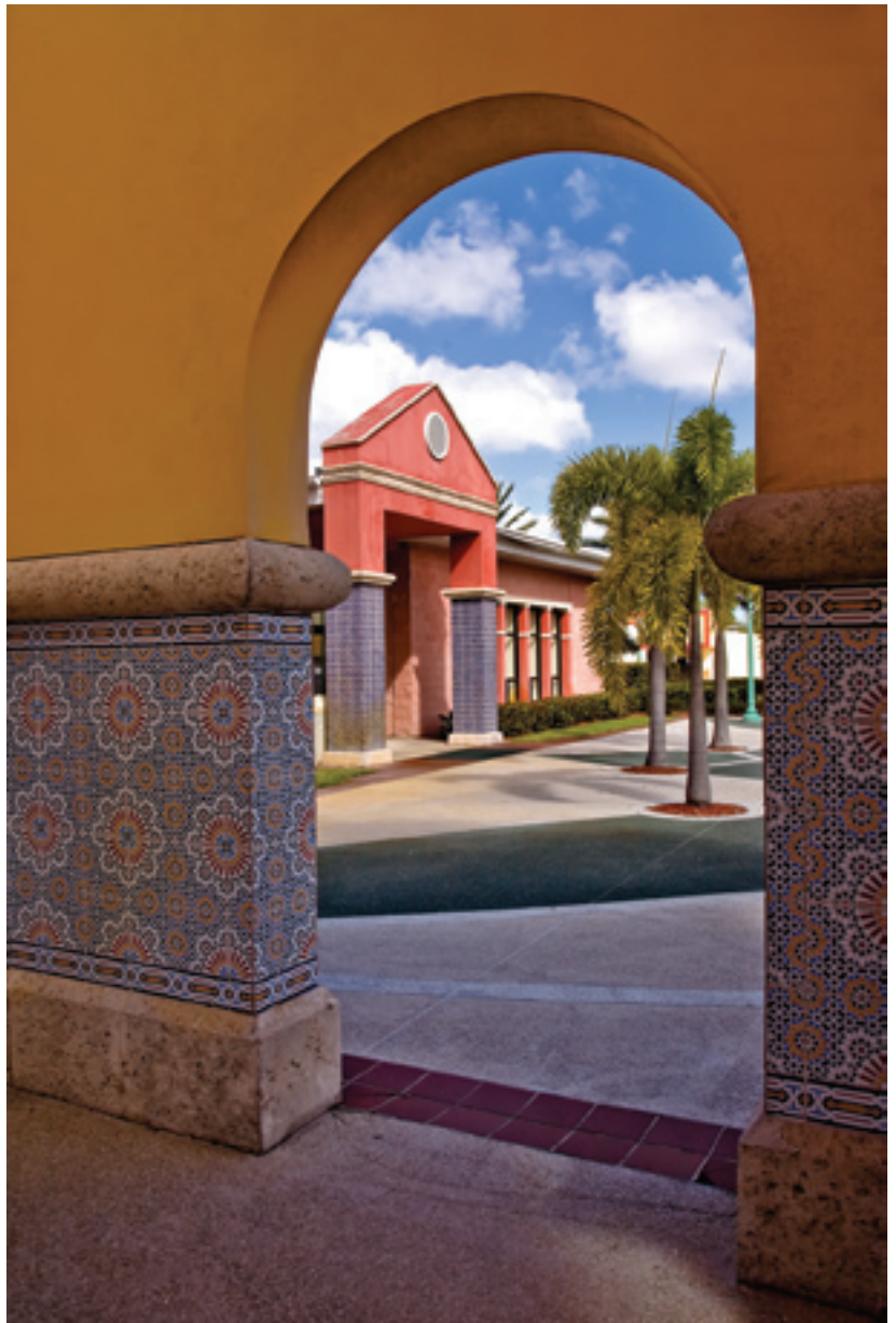
Community Building Arch to Courtyard
