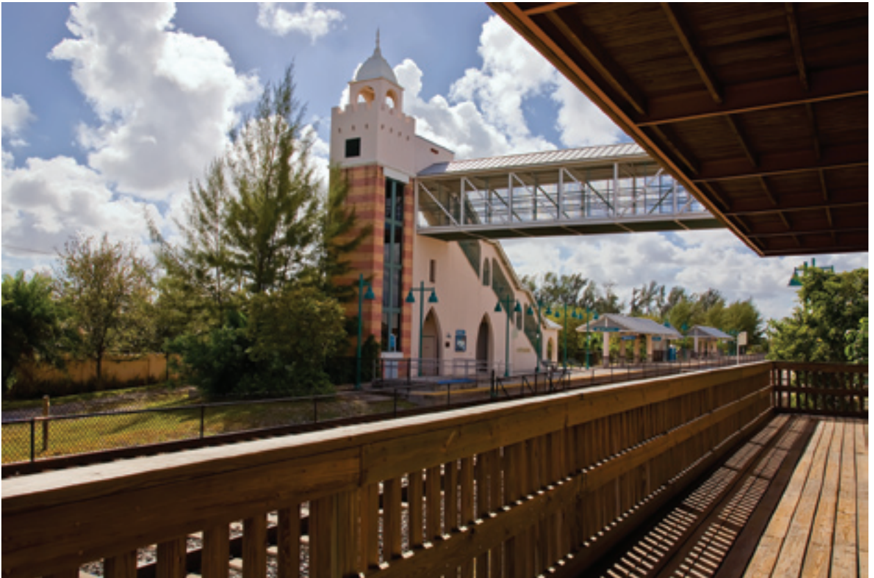
Train Station new construction
