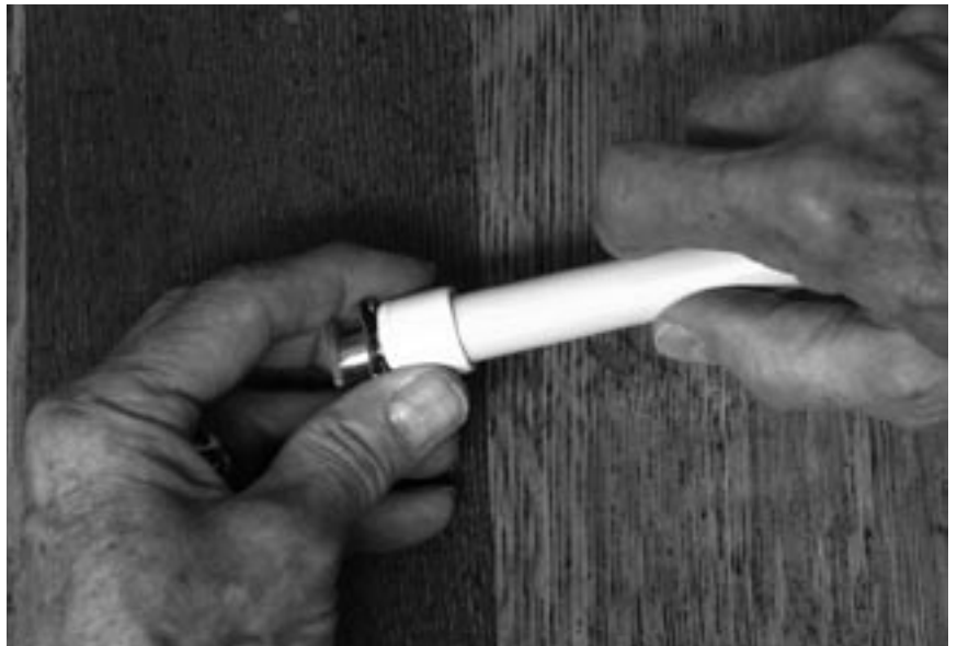
Insert PVD pipe into cap
